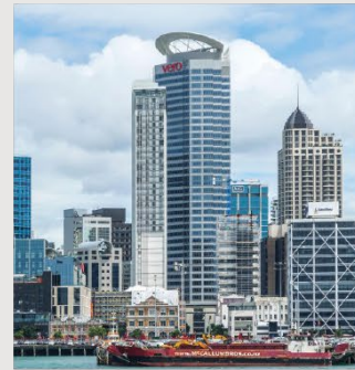
Vero Tower (Centre) 2000 48 Shortland Street Peddle Thorp + Walker – Office – 170.3m / 39 Storeys – Tower diagonal: 45m aprox. – Site Area: 4,426m 2
