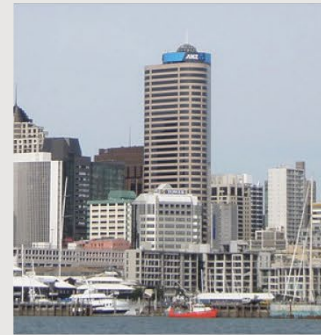
ANZ Centre 1991 23-29 Albert Street Hassell – Office – 159m / 37 Storeys – Tower diagonal: 42m aprox. – Site Area: 3,295m 2
