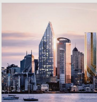
Seascapes 87 Customs Street East Peddle Thorp Architects
